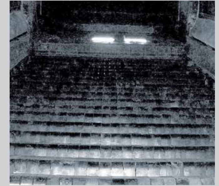
Grate bars in waste incineration
